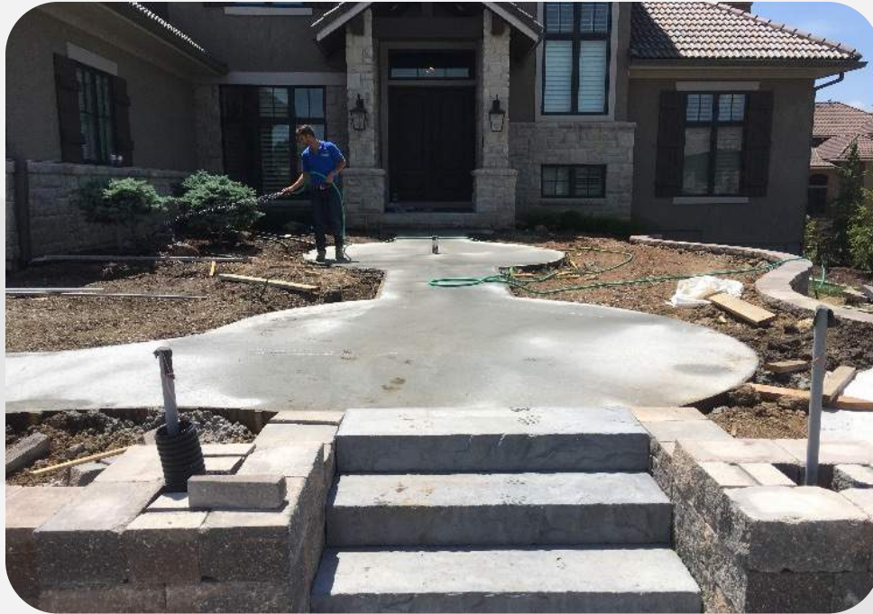
This picture above shows what AB-3 looks like after being compacted.
