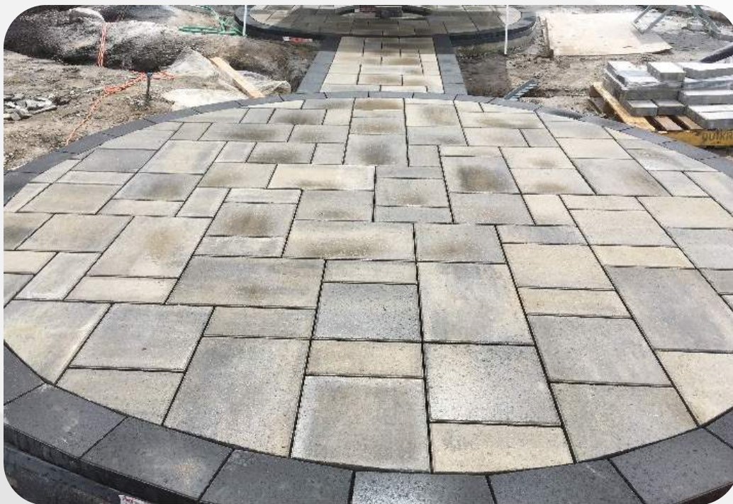
This picture shows the pavers prior to sand being installed.
